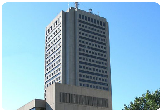
Photo: Marie-Guyart building in Québec City, offices of the ministère de l'Éducation Source: Gilbert Bochenek (2007) via Wikimedia Commons, Public Domain c
